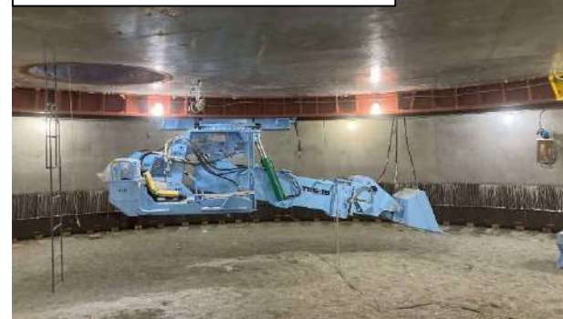
④掘削・沈設
